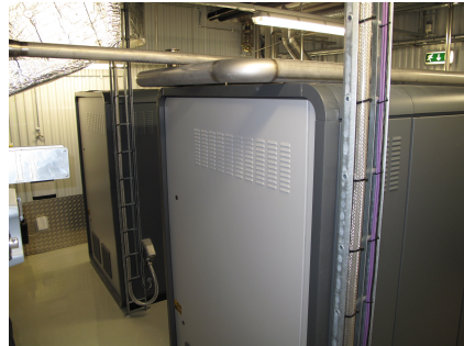
(b) Air-to-water intercoolers.
