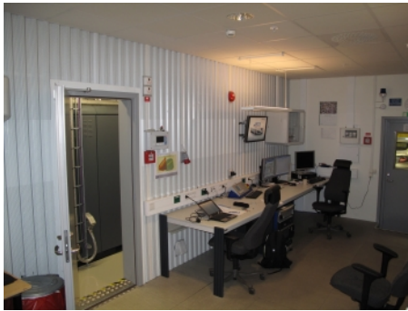
(c) Control room
