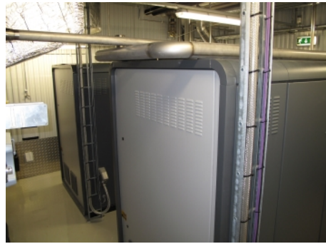
(b) Screw compressor room.
