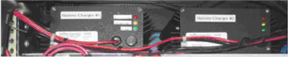
**Figure 3.8.** Picture of the battery charger panel containing the two battery chargers taken from [17].
