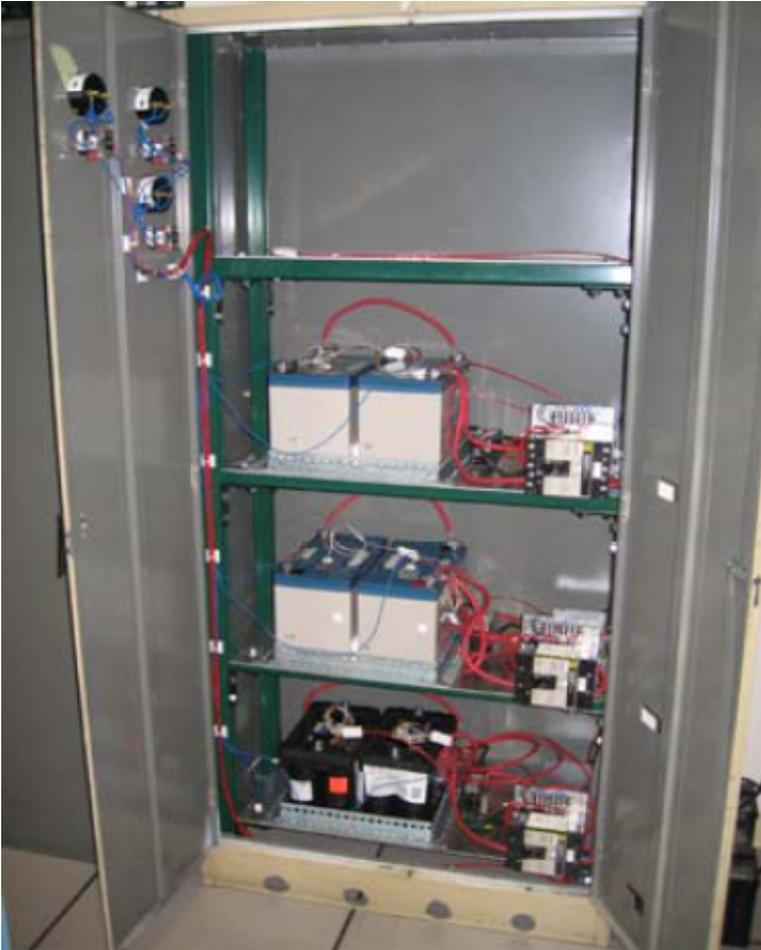
**Figure 3.5.** Picture of the battery cabinet with the three battery packs inside taken from [17].
